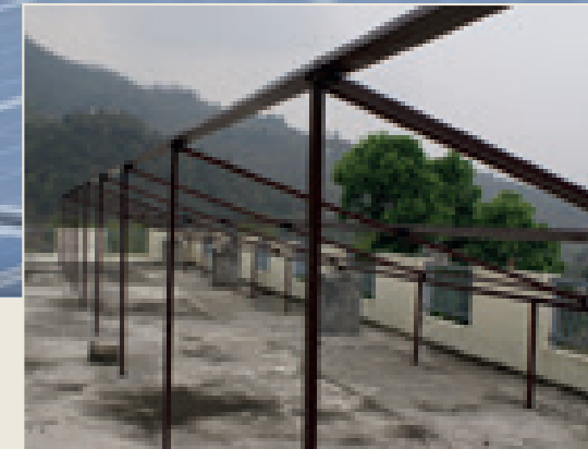
Steel construction for the solar panels
