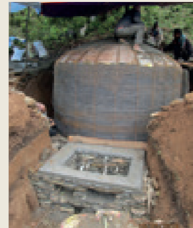
Tangle construction site: water tank and connections
