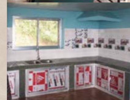
The work on the health Post, finished interiors and helipad
