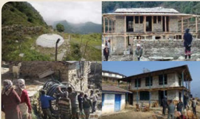
Far left: Water storage tank, laying of pipes Left: Building of the youth club Below: School building
