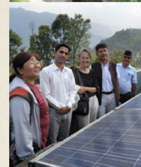
The team during the visit: Laxmi, Ganesh, Christina, Raj, Tanka. Impressive: the photovoltaic system on the roof of the Himali school in Bhakunde
