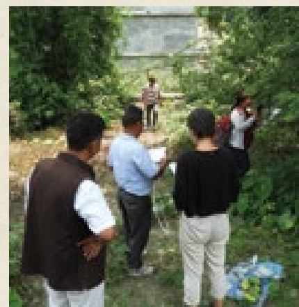
Inspection and measurement of the building site for the Mustang House
