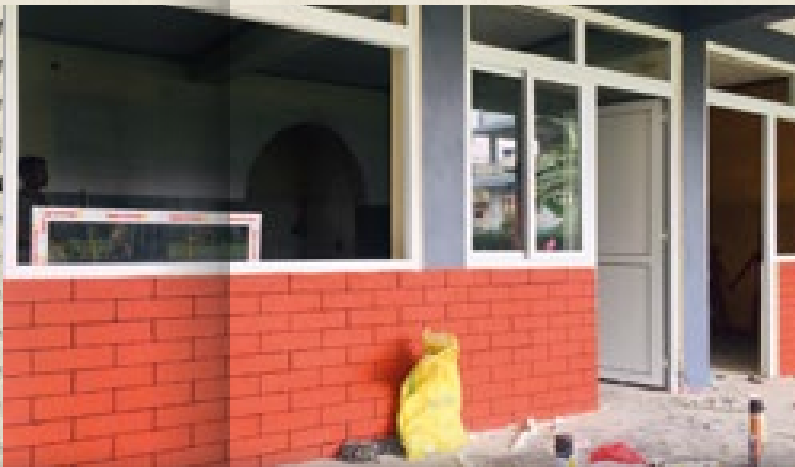
The reconstruction work has begun
